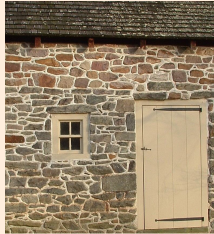
Detail-Valley Forge building
